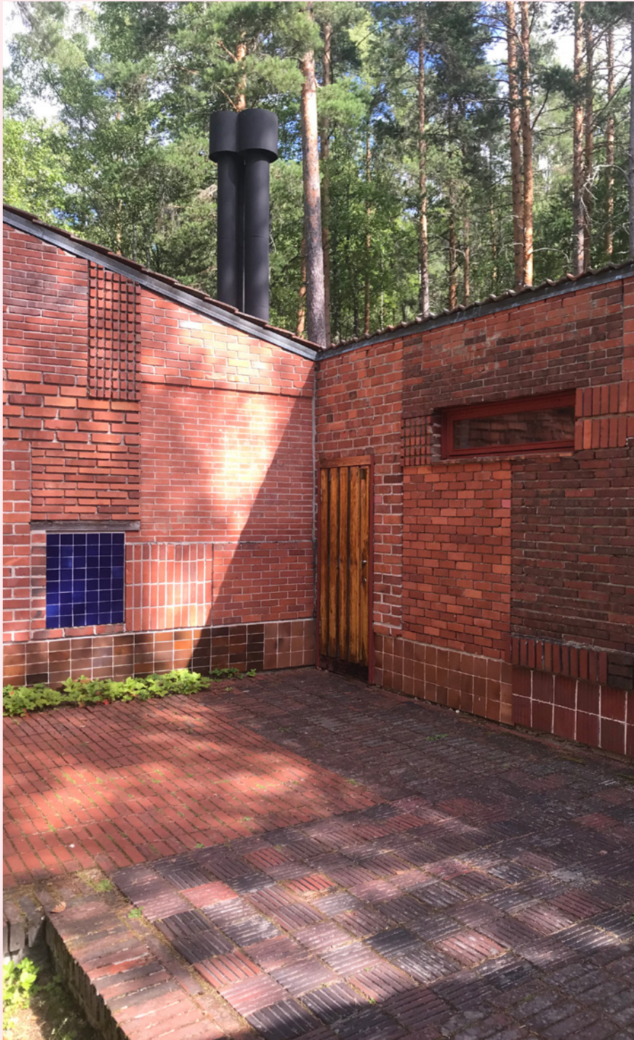
The Muurtasalo Experimental House 2020. After the restoration of the patio. The bricks were laid back in the same manner they had been originally. Photo: Tommi Lindh.
