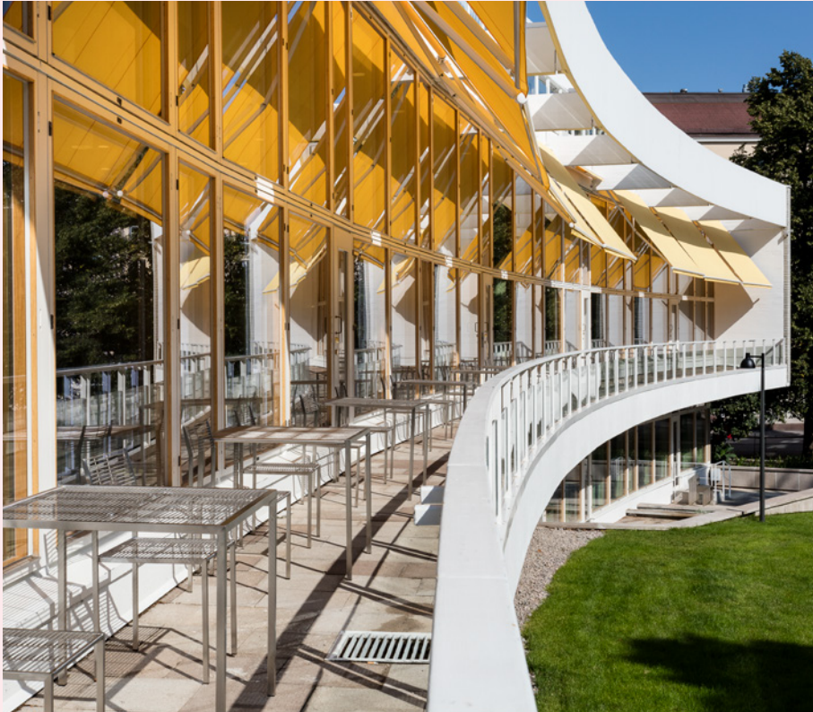
The Töölö Municipality Library 2016. Balcony after renovation. Photo: Architects Mustonen.
